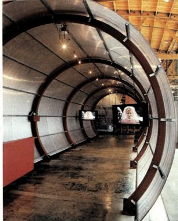
OGILVY & MATHER | Perforated aluminum sheet panels make up the entryway, a.k.a. the Tube, that leads to the main work area.
